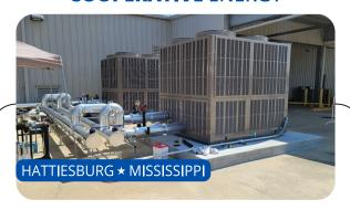
Metro Mechanical recently completed work at the headquarters of Cooperative Energy in Hattiesburg, Mississippi. Work included removal of geothermal water source heat pumps and installation of two 50-ton chillers and associated piping. This member-owned electric cooperative serves over 432,000 homes and businesses in 55 of Mississippi's 82 counties. With history dating back to 1941, South Mississippi Electric was renamed Cooperative Energy in 2016.
